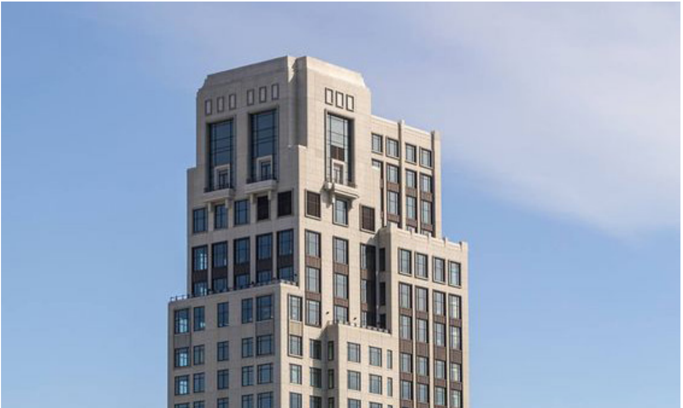
Figure 20: This mechanical penthouse is fully integrated with the architectural expression to create a dynamic skyline profile.
