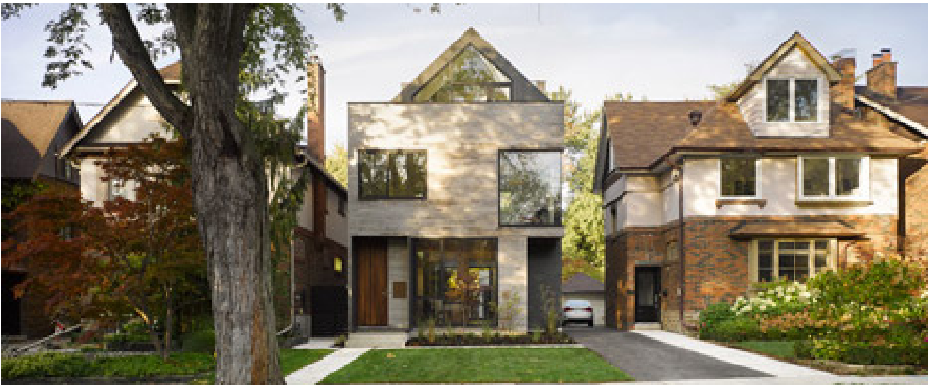
Figure 55: The new dwelling, while modern, references many characteristics of the existing buildings along the streetscape including massing, setback, prominent entry, and roof form.
