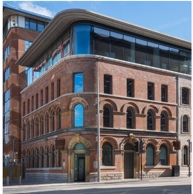
Figure 45: Taller components of new development are stepped back from the primary heritage facade.
