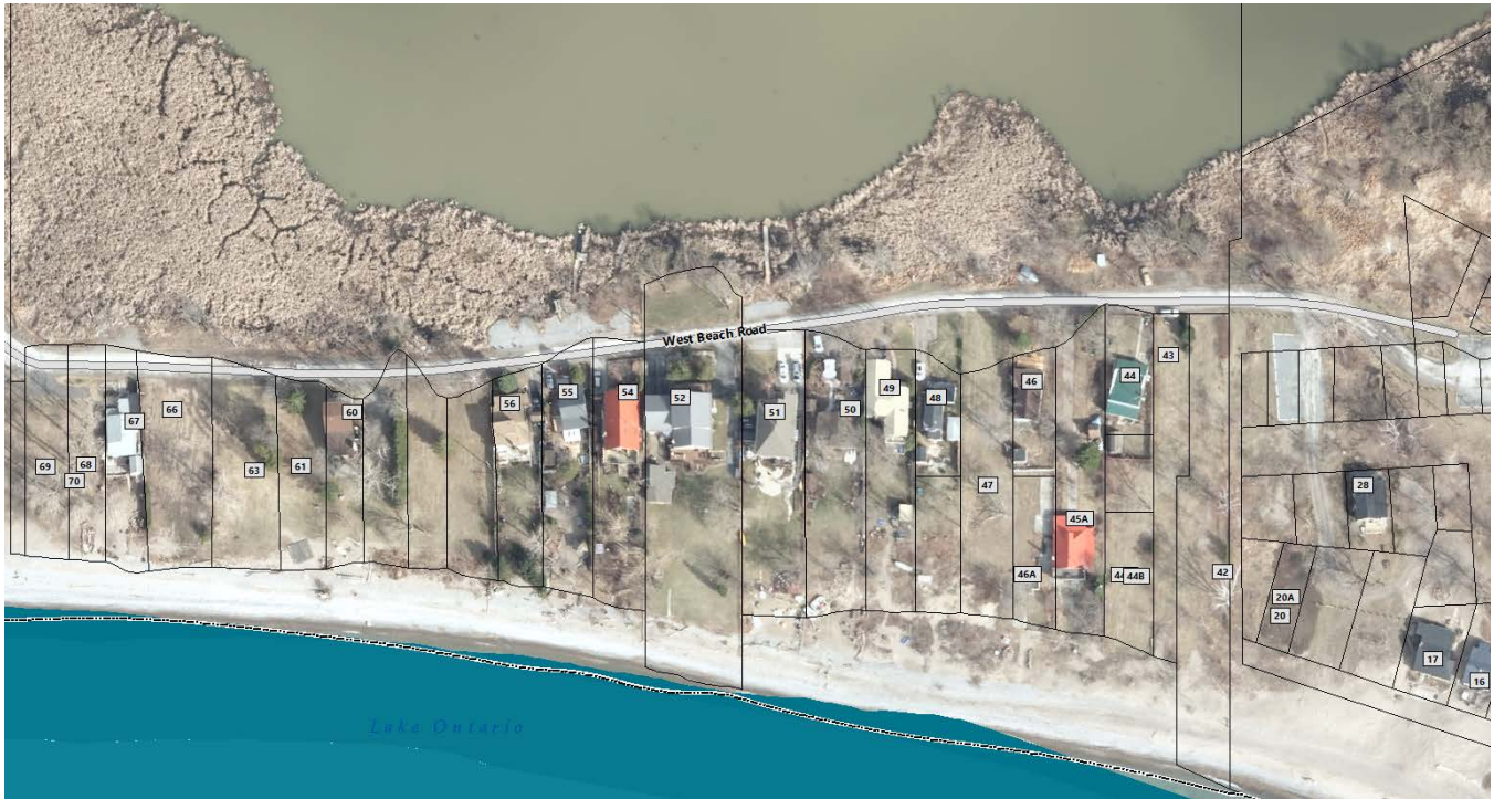
Figure 5: Property Limits and Marsh Along West Beach Road
