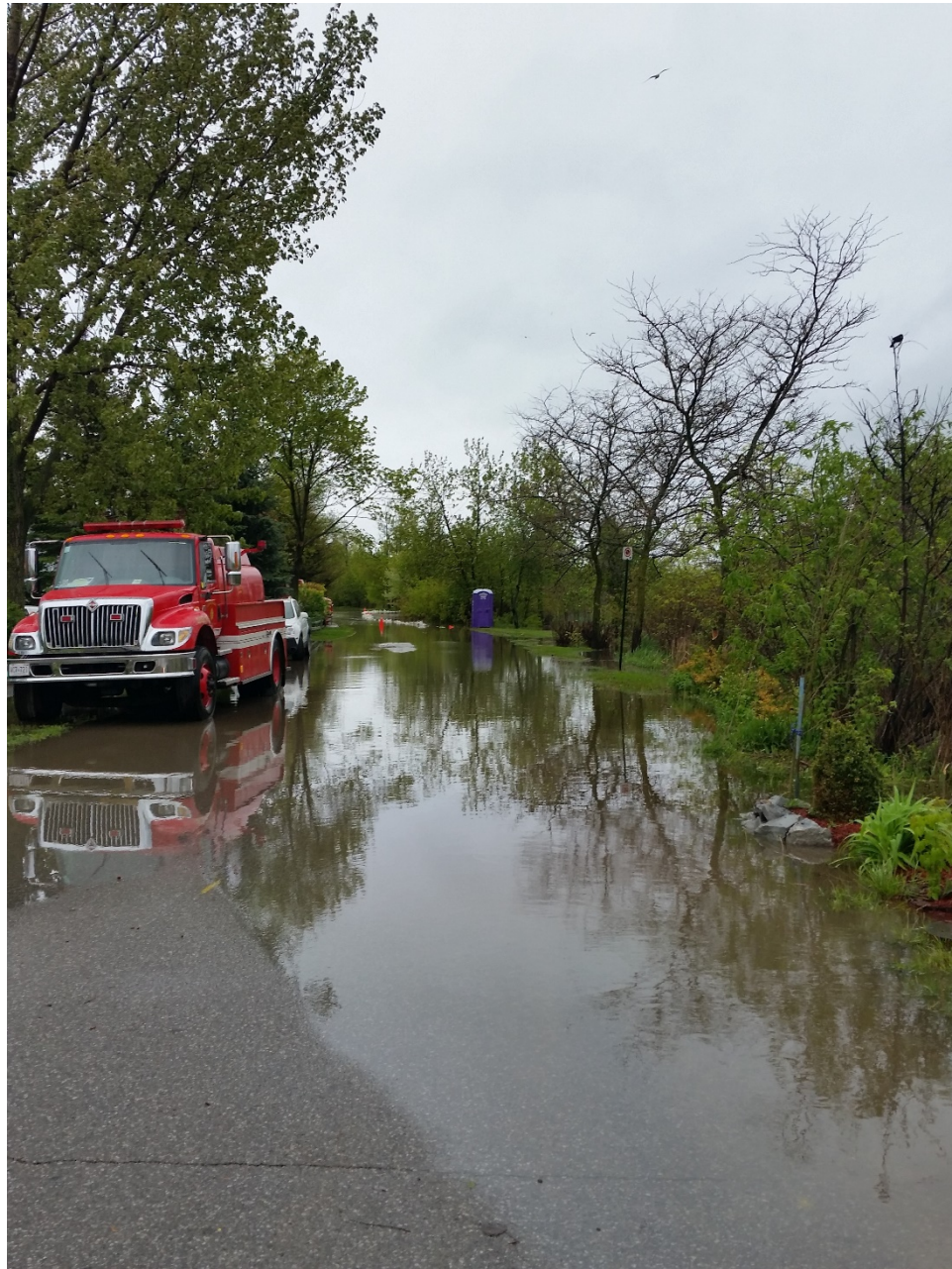
Figure 2: Cedar Crest Beach Road Flooding
