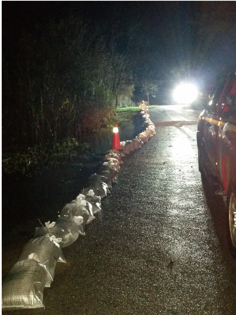
Figure 3: Sandbag Berm on Cedar Crest Beach Road
