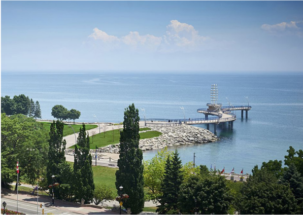
PIER IN BURLINGTON, ON
