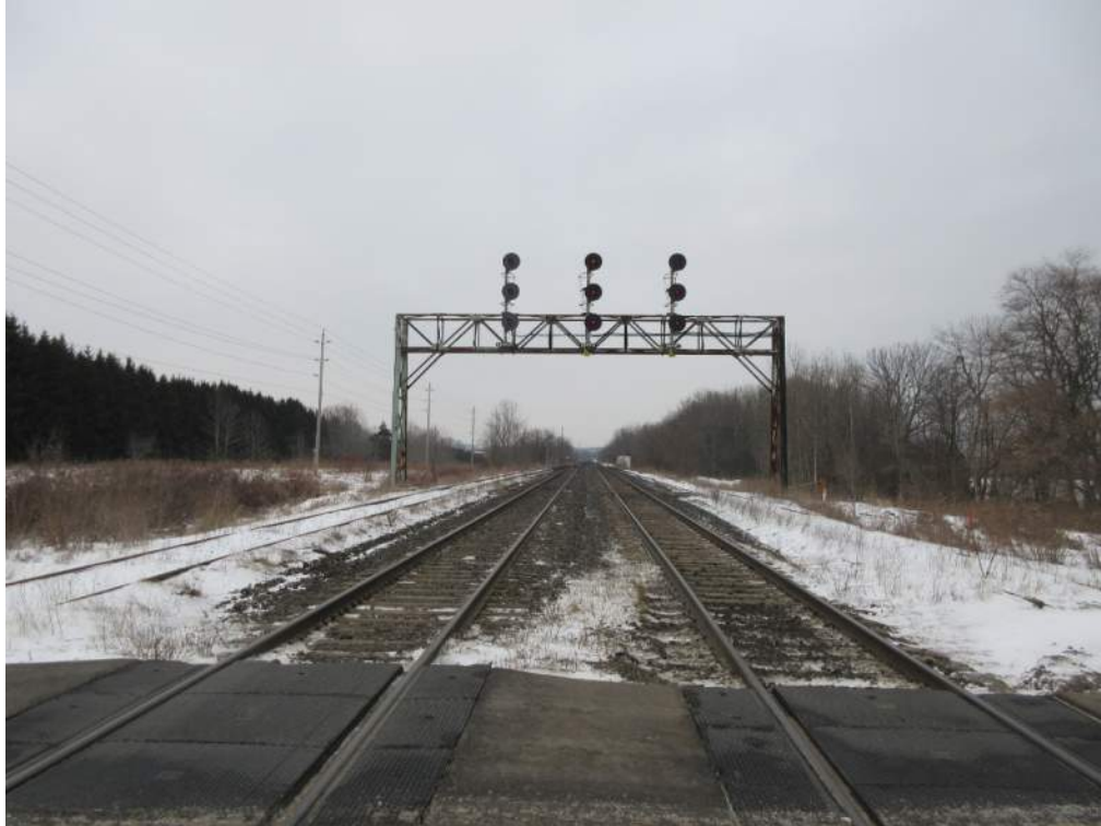
Photo 3: Rail approach, looking east.
