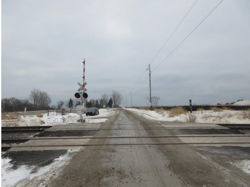
Photo 5: Road approach, looking south.
