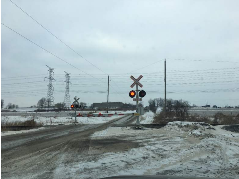
Photo 27: Front light units on the south road approach aligned towards intermediate areas on the south east quadrant.
