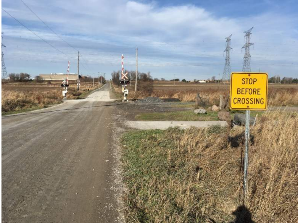
Photo 23: “Stop Before Crossing” sign placed along south road approach, east side of road.
