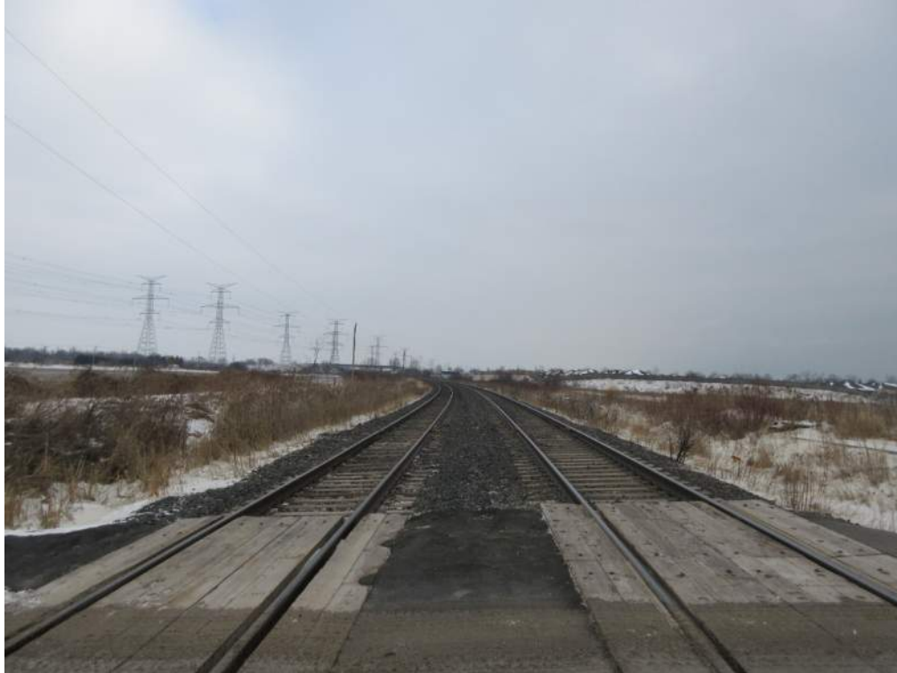
Photo 1 – Bennett Road crossing, rail corridor looking east.
