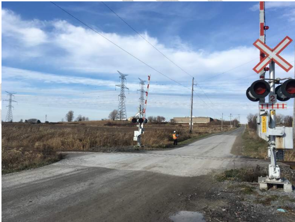
Photo 18: Property access on south road approach, east side, 5m from crossing.
