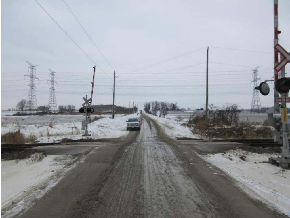
Photo 1: Road approach, looking north.
