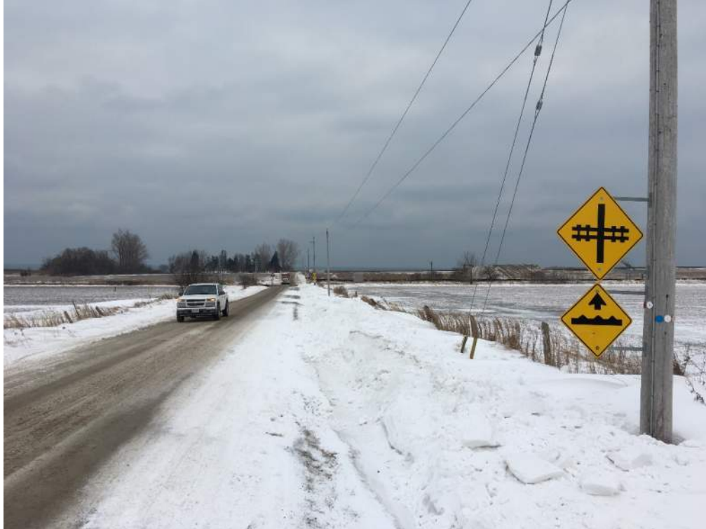
Photo 29: WA-18 sign, WA-22 sign placed on same pole on north road approach.
