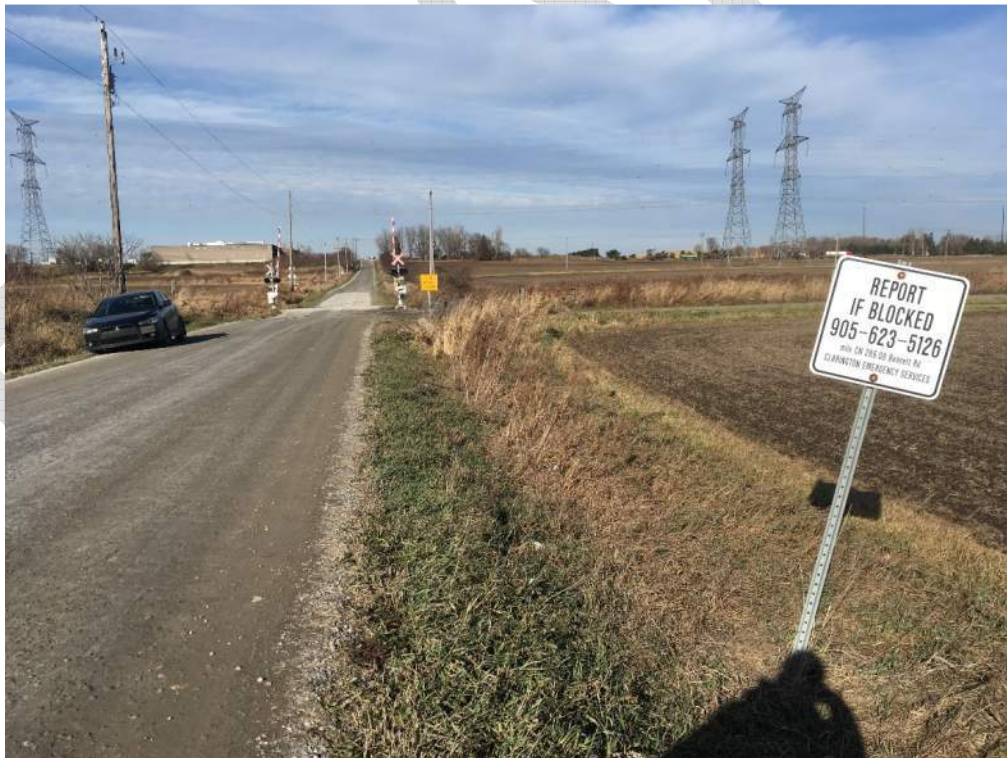
Photo 24: “Report if Blocked...” sign placed along south road approach east side of road, sign is leaning eastward.
