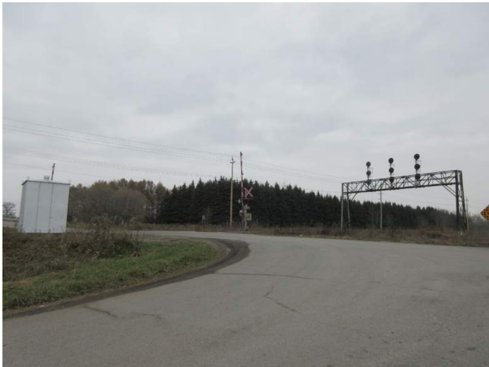
Photo 14: Service Road and Cobble Dick Road intersection, 20m from crossing along south road approach, west side. Back lights obstructed by Warning System Housing Unit on south west quadrant. No stop bar present on Service Road at stop sign.
