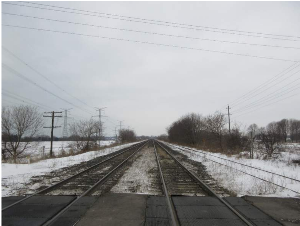
Photo 4 – Cobbledick Road crossing, rail corridor looking west.
