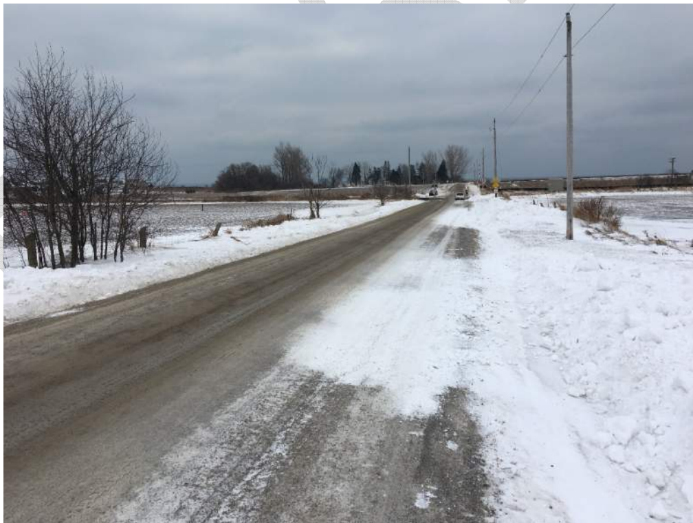
Photo 28: North road approach, crossing at SSD of 110m for road speed of 50km/h. "X" pavement markings are not present.
