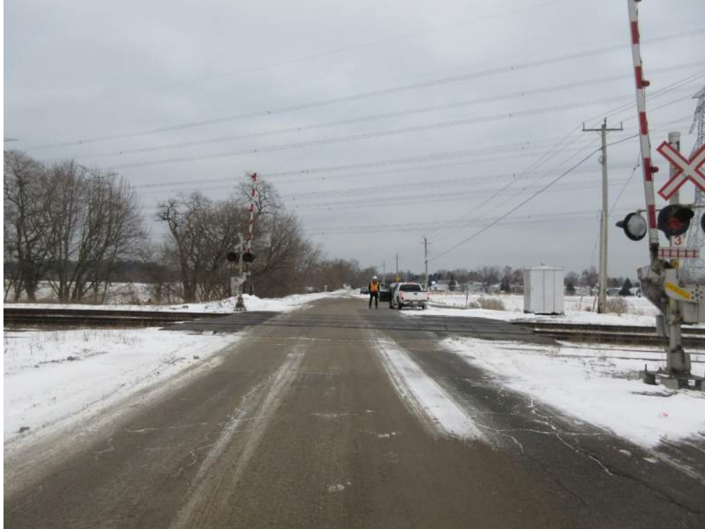
Photo 5: Road approach, looking south.
