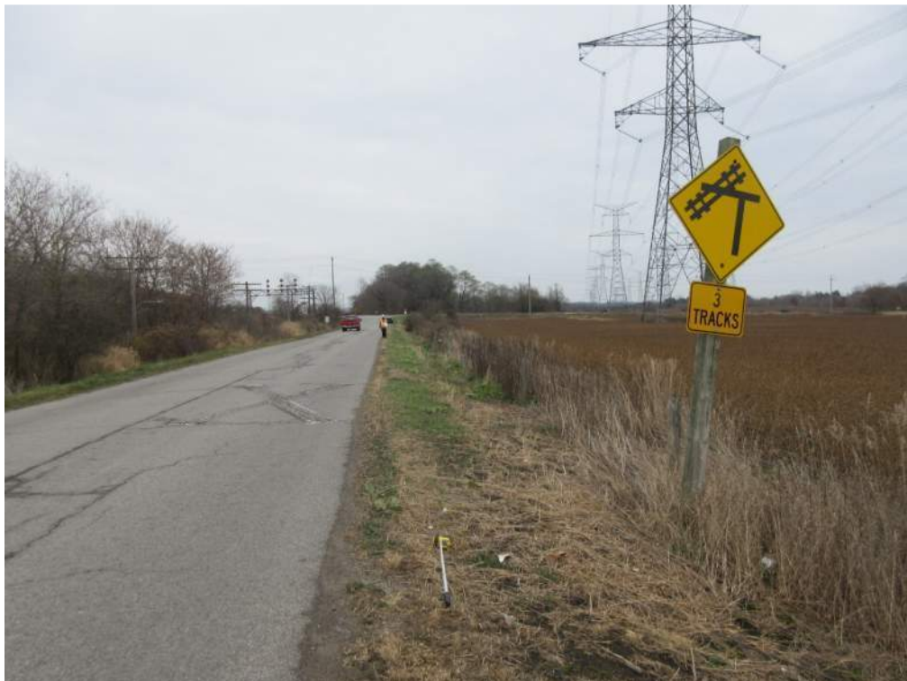
Photo 24: Modified WA-18 sign on Service Road located 168m from Cobble Dick Road intersection. Sign does not depict accurate track angle configuration and number of tracks.
