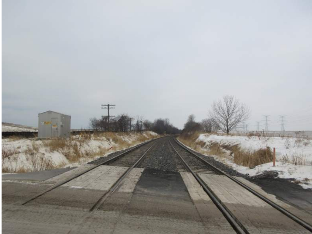
Photo 7: Rail approach, looking west.
