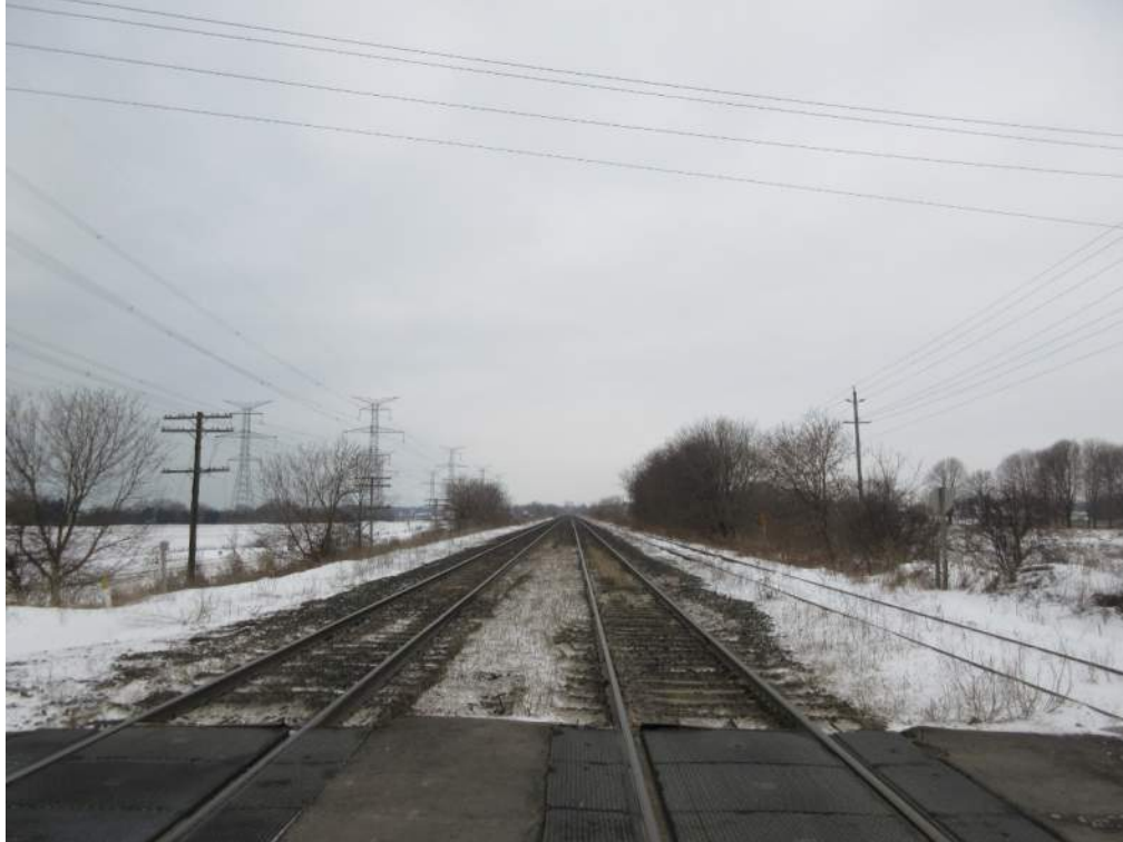
Photo 7: Rail approach, looking west.
