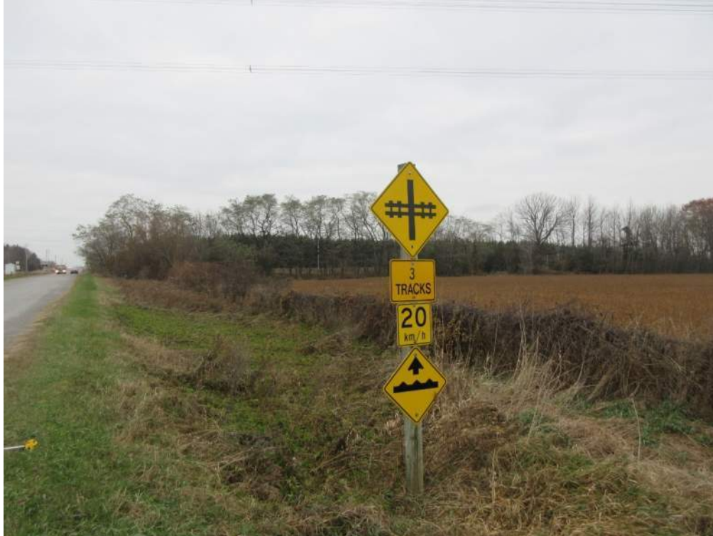
Photo 17: WA-18, WA-22, Advisory Speed Tab sign and “3 Tracks” sign placed on the same post located beyond 110m on the south road approach. Sign is also located in a ditch and the WA-22 sign may not be visible from certain angles on the road. WA-18 sign does not show correct number of tracks.
