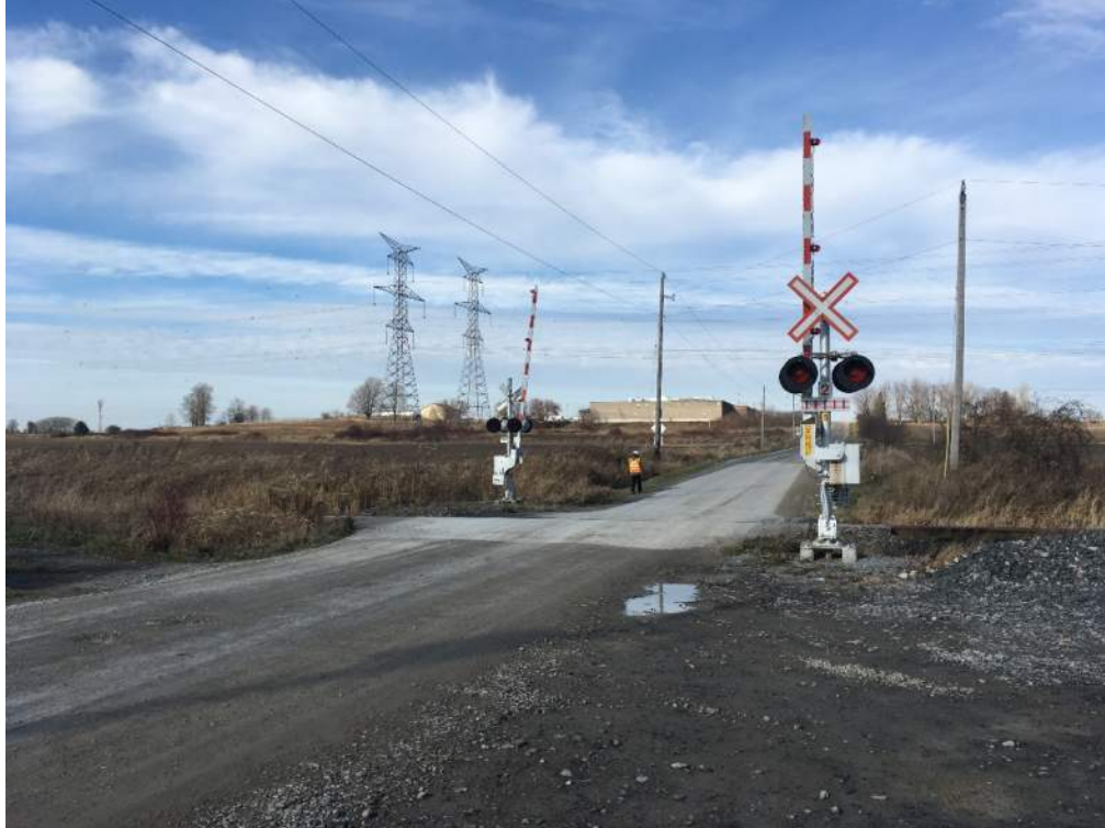
Photo 19: Property access on south road approach, east side, 14m from crossing.
