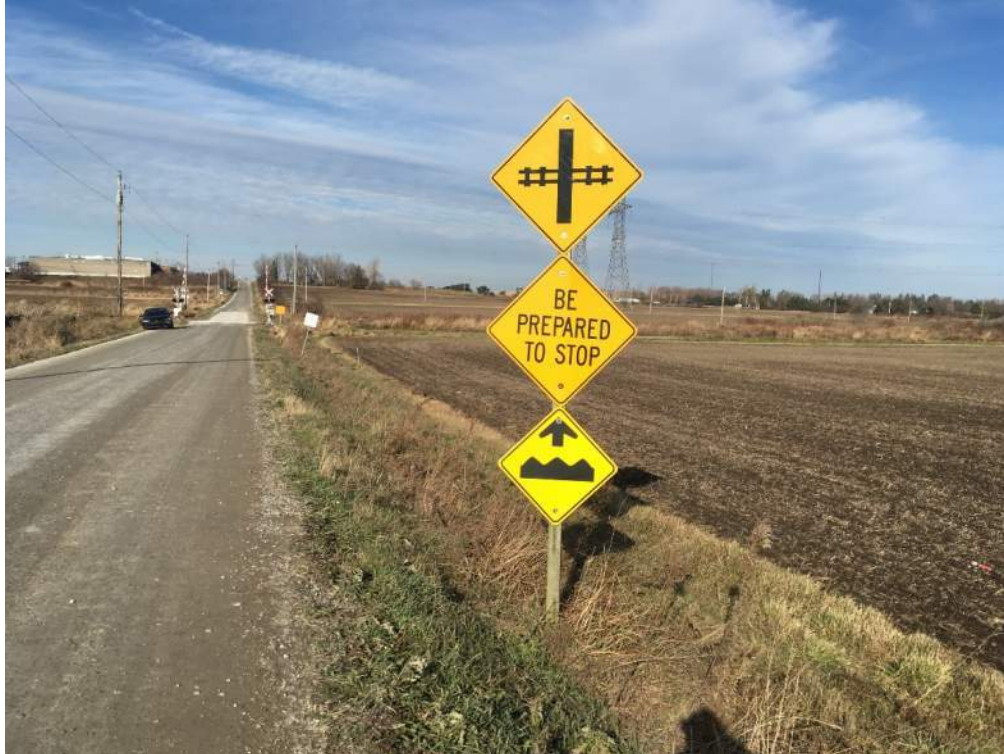
Photo 25: WA-18 sign, WA-22 sign and “Be Prepared to Stop” sign placed on same pole on south road approach. Signs are not aligned perpendicular to the road.
