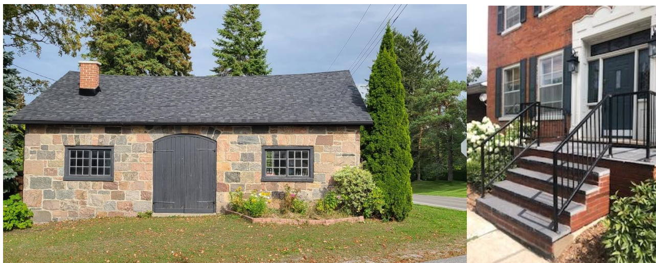
Figure 1: Completed works at 2752 Concession Road 7 and 67 Ontario Street
